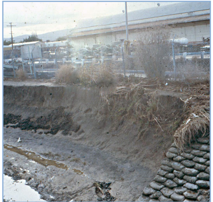
Erosion along the Sunnyvale East Channel
