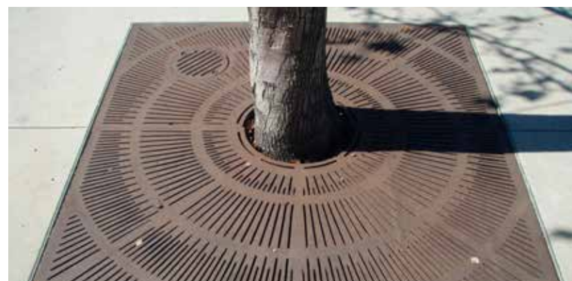
Installed correctly, large tree grates provide increased sidewalk pedestrian space, a larger growing area, and additional water and air to tree roots.
