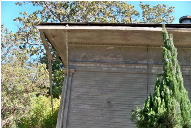
21. Exterior wood trim is in a highly degraded condition and absent in some locations.
