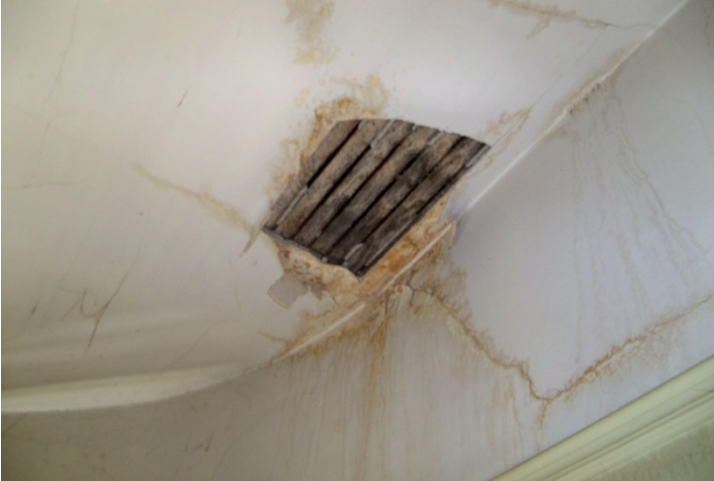
31. Evidence of roof leaks was observed in several locations.
