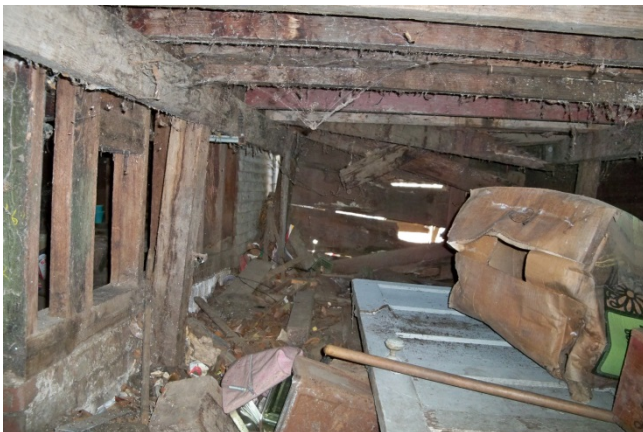
23. Wood framing underneath back porch is in a highly degraded condition and is structurally unsound.
