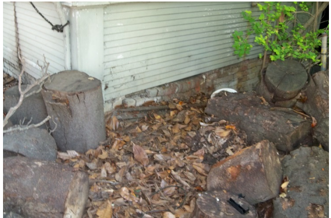
28. Non-reinforced brick masonry pony walls are in a highly degraded condition with evidence of subsidence observed.
