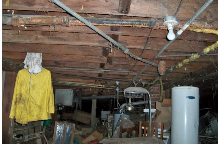
38. Electrical wiring and piping, both for gas and water service, are presumed to date to original construction.
