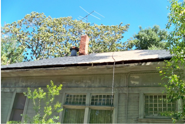
19. The asphalt composite shingle roof is in a highly degraded condition.
