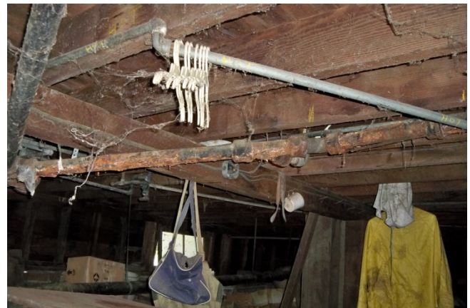
24. Typical condition of wood framing in crawlspace. Cast iron drain piping is heavily rusted in various locations.
