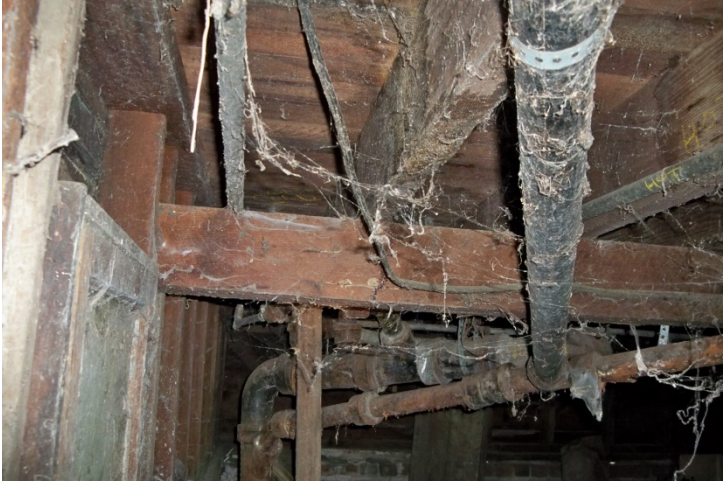
37. Electrical wiring and piping, both for gas and water service, are presumed to date to original construction.
