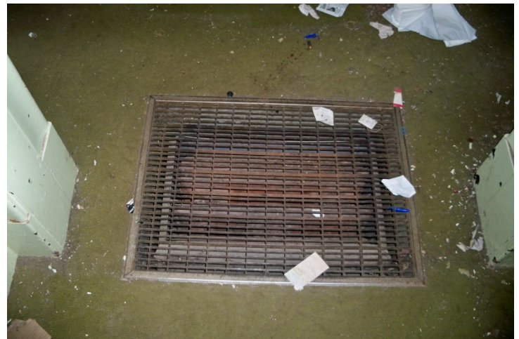
36. A natural gas-fired floor furnace, presumed to date to original construction, is installed.
