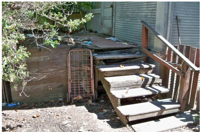
6. Degraded condition of rear stairs and back porch.
