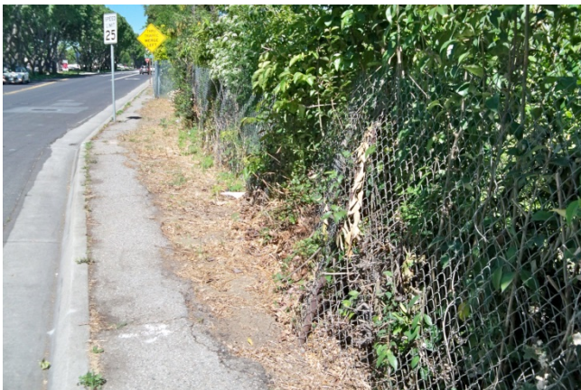
17. Various portions of the fence have out of plumb posts and bulging chain link.
