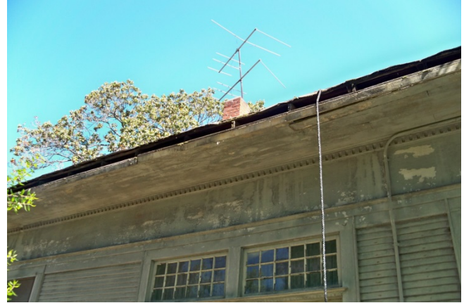
20. Soffits, fascias, gutters, and downspouts are in a highly degraded condition. Gutters are missing altogether in several places.
