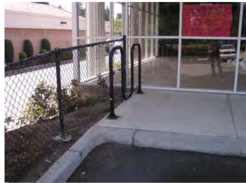
d) U-lock-capable rack, siting prevents use
