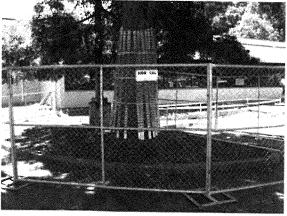
The protective fencing must not be temporarily moved during construction. Materials, tools, excavated soil, liquids, substances, etc. shall not be placed or dumped, even temporarily, inside the RPZ. Storage, staging, work, or other activities shall not occur inside the RPZ without the expressed written (emailed) permission from the assigned project arborist.
