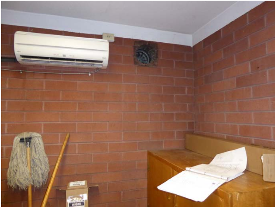
Photo 11: Hole in exterior brick masonry wall in UPS room.
