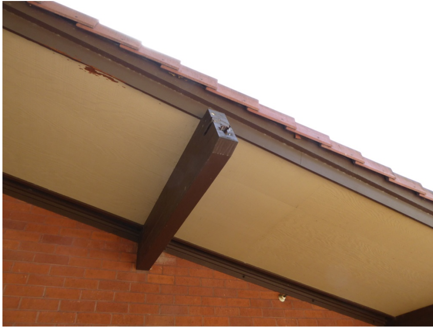
Photo 19: Damaged exterior roof beam.
