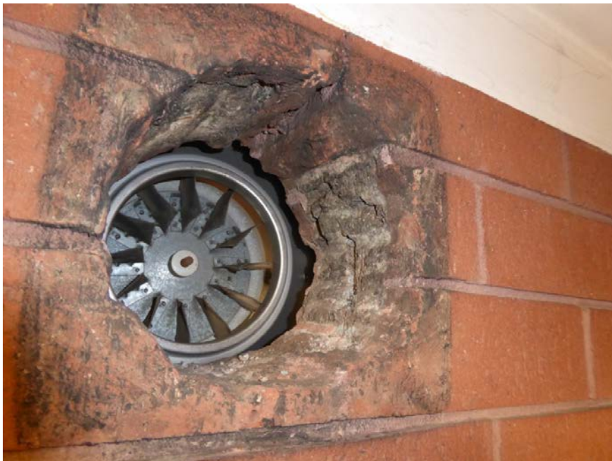
Photo 12: Hole in exterior brick masonry wall in UPS room.
