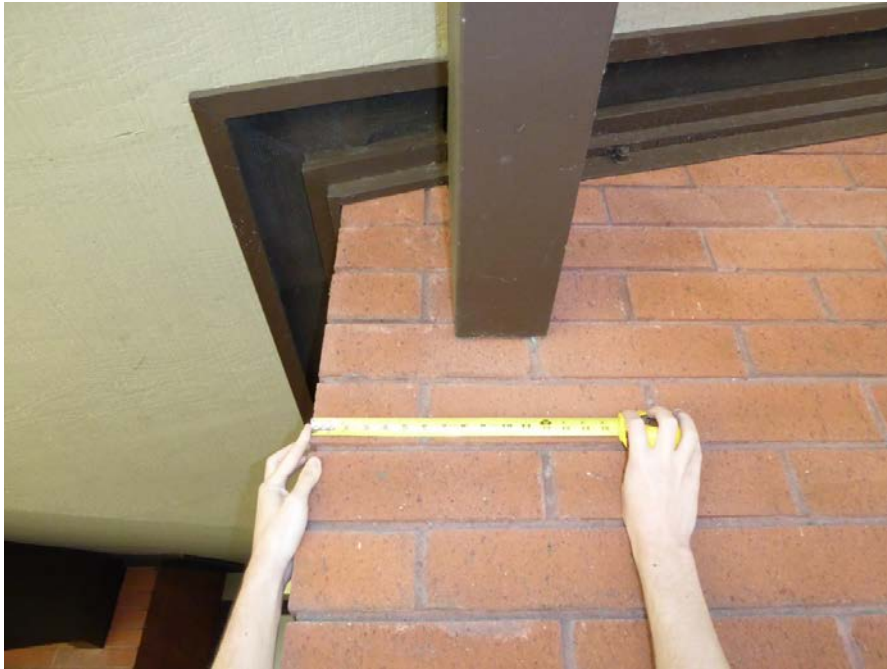
Photo 15: Glulam beam at exterior brick wall corner.
