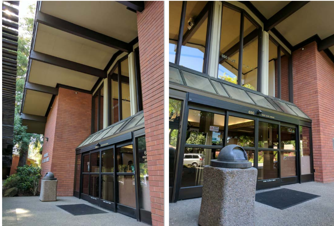
Figure 3: Existing Building Entrance
