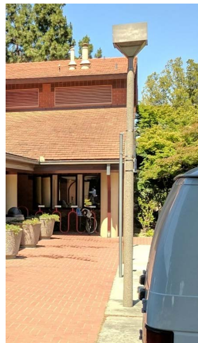
Figure 41: Typical Exterior Light Fixtures
