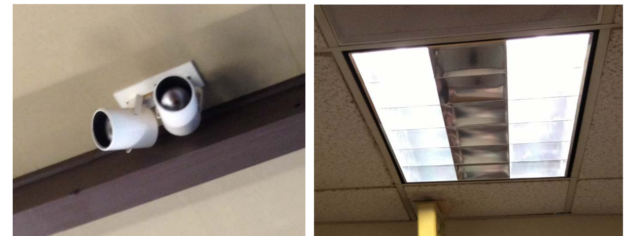
Figure 23: Typical Interior Light Fixtures
