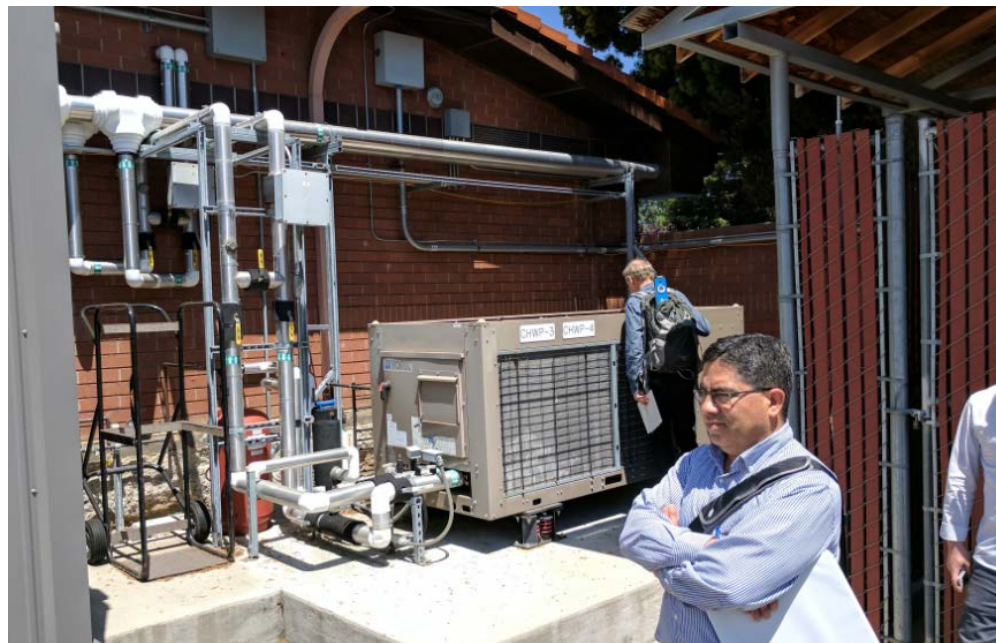
Figure 31: Annex Building HVAC Controls Panel
