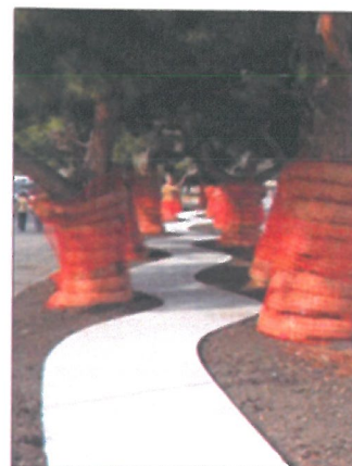
Photo 3: Protect trunks of trees by winding silt sock wattle and orange snow fencing around trunks.
