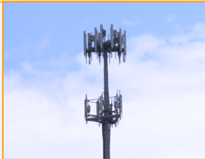
Typical Macro facility – industry standard sized colocateable facility with full compliment of radios
