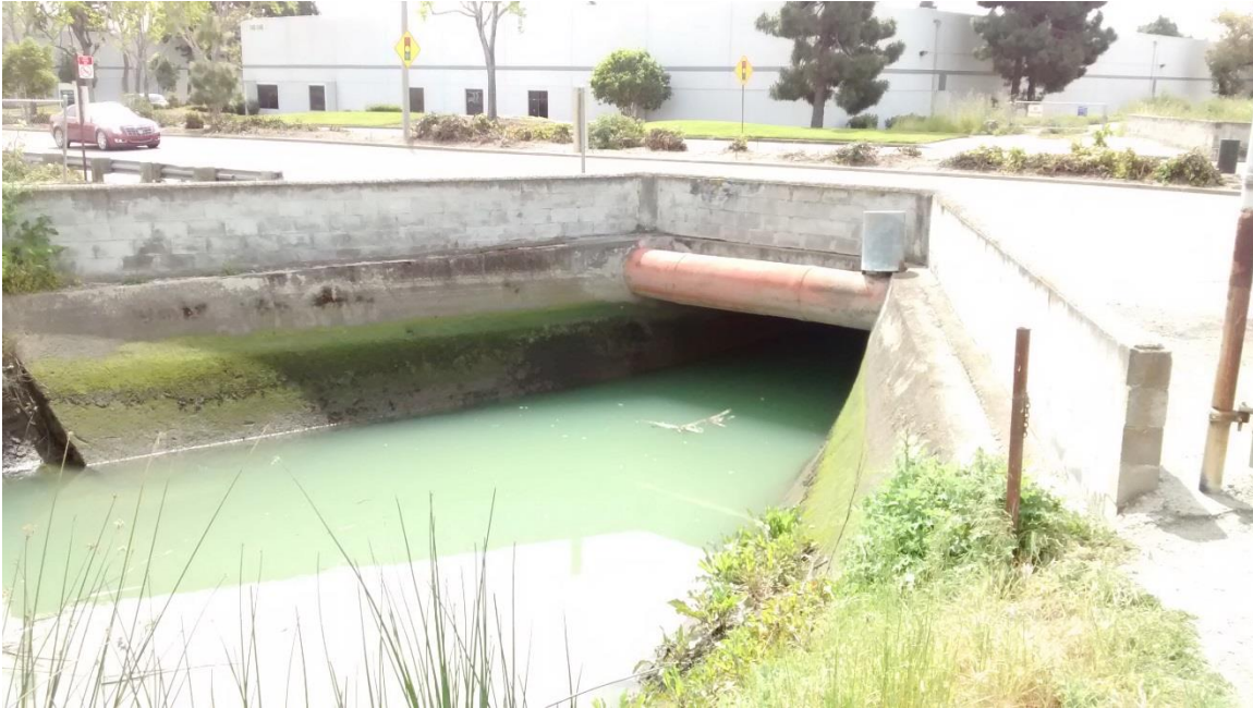
Sunnyvale West Channel headwall at Caribbean Drive
