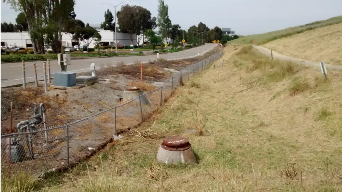
Looking west down Caribbean Drive at headwall
