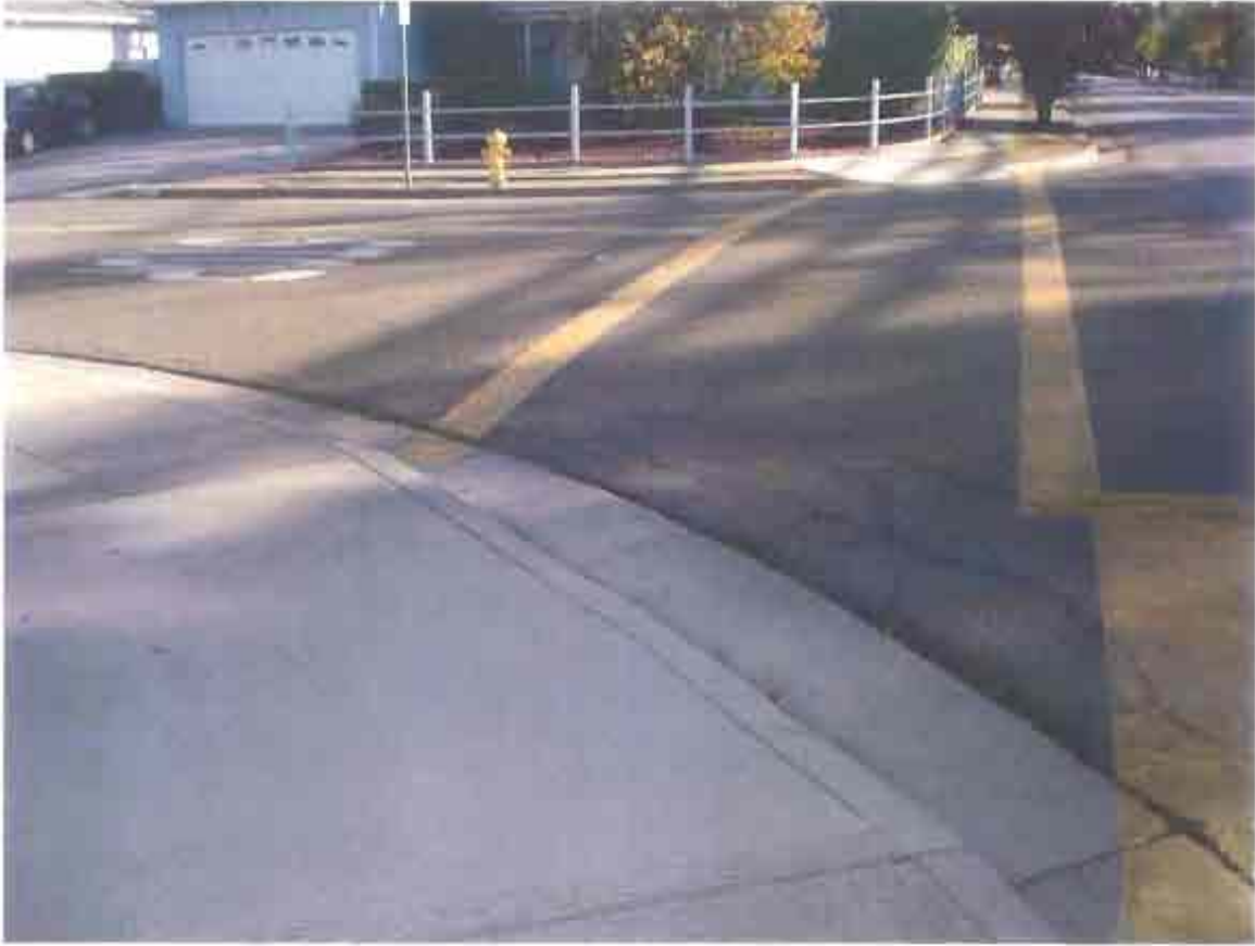
Marked School Crosswalk
