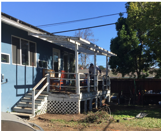
Original deck and pergola before demolition (early 2018). Structural compromise is evident as 'sagging' and boards were rotted out creating a safety hazard.
