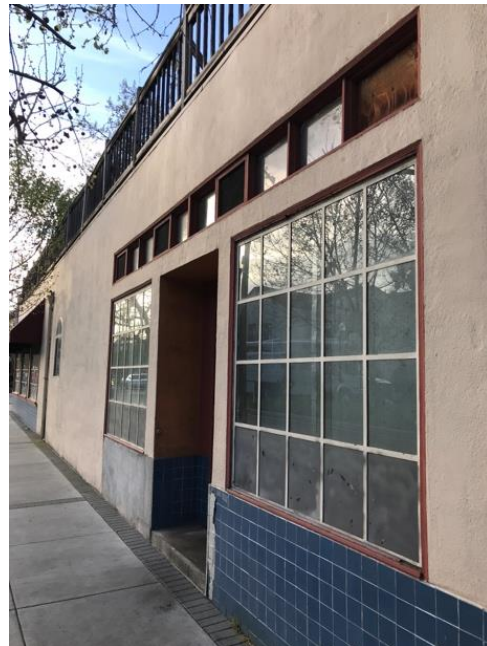
Below: Evelyn Avenue showing missing tile and need for transom window restoration.
