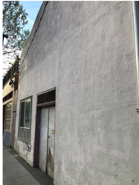
Above: View of required repairs to stucco, windows and doors at the Evelyn Avenue façade.
