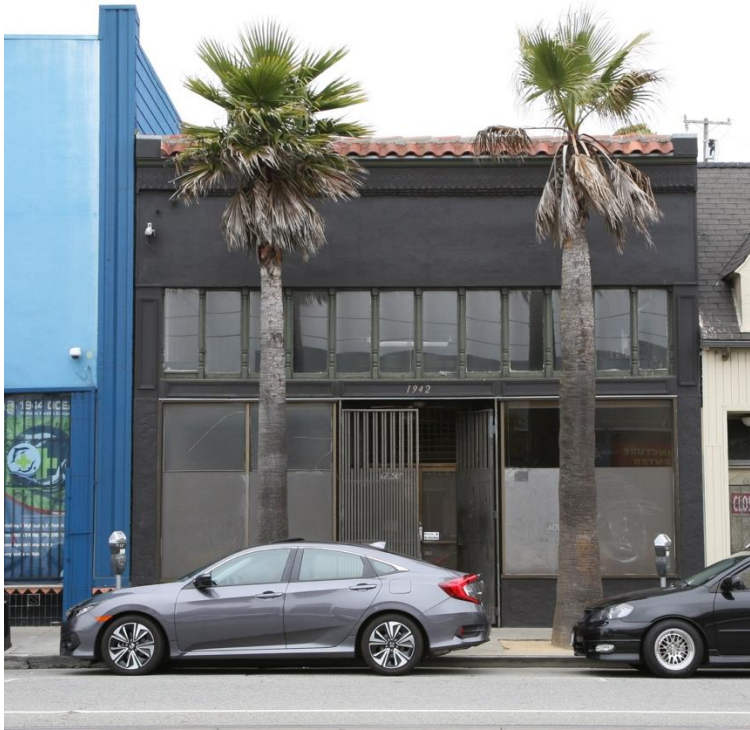
Above: This storefront was intact at the upper level but had been badly remodeled at the lower portion of the storefront. Recently, it was remodeled again with large panes of glass, a recessed entry with nicely designed gate, and a simple, but solid base. It blends well with the other historic storefronts on the street.
