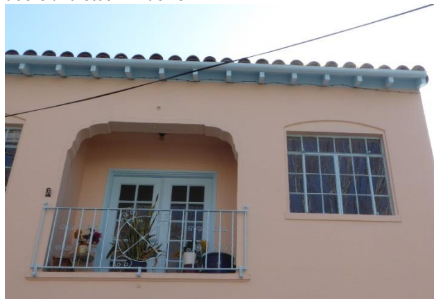
Below: Upper level balcony with railing and wood double doors and steel windows.
