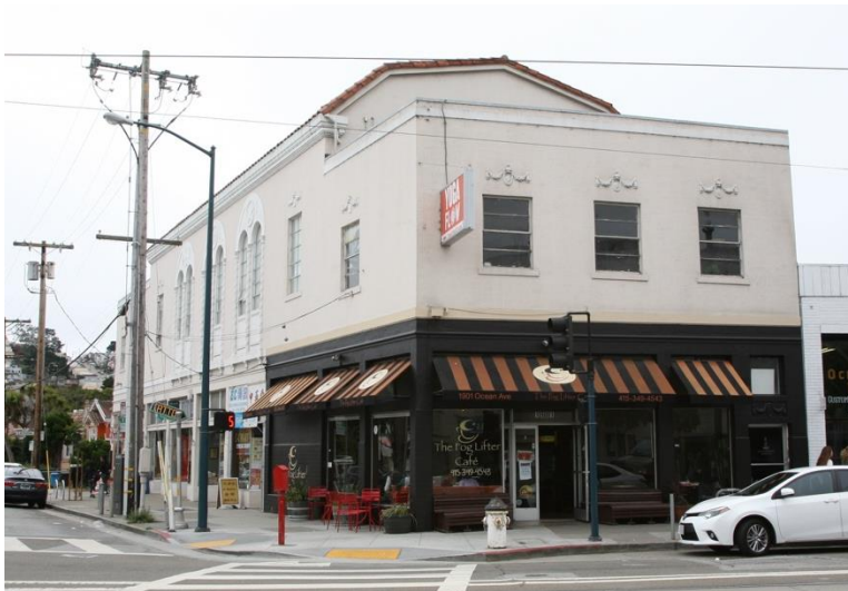
Above: This is a good example of using several awnings of the same size and character along a corner storefront to break up the awning plane and highlight the individual elements of the building.
