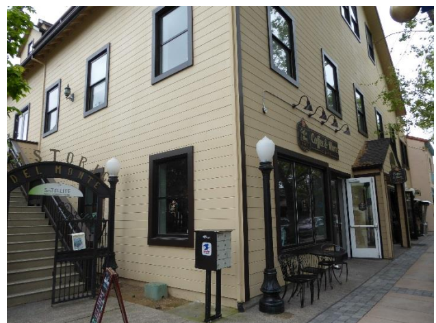
Corner of building, with double hung windows.
