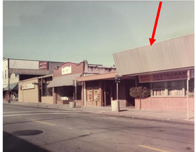
Above: Historic photograph showing original configuration of the front façade.
