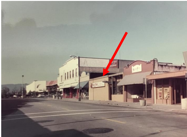
Below: Historic view of the building before significant alterations.
