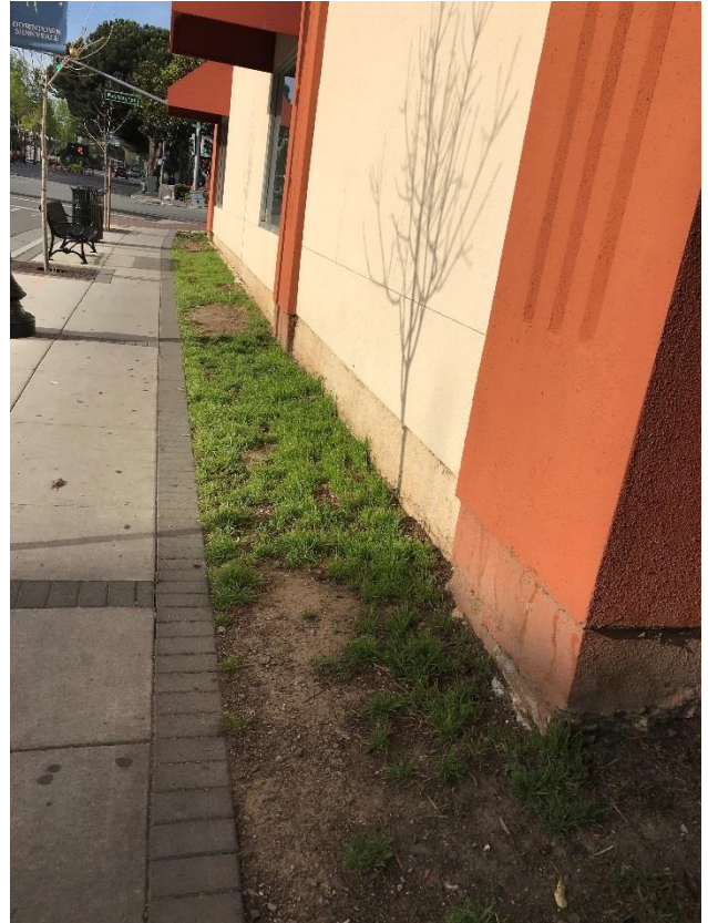
Above: S. Sunnyvale elevation showing planting area between building and sidewalk.
