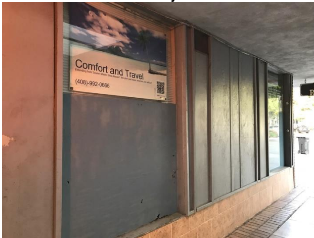
Below: Wall within the breezeway.
