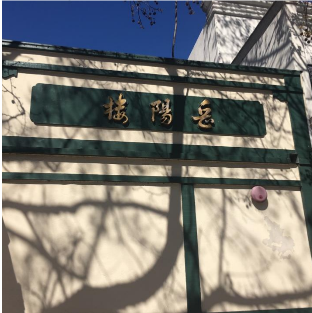
Above: Detail of the north end of the front facade
