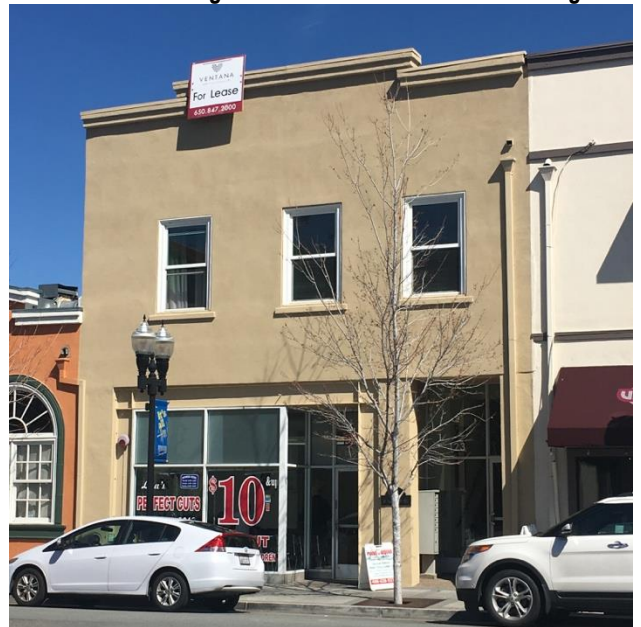
Below: The Washington Street elevation of the building.
