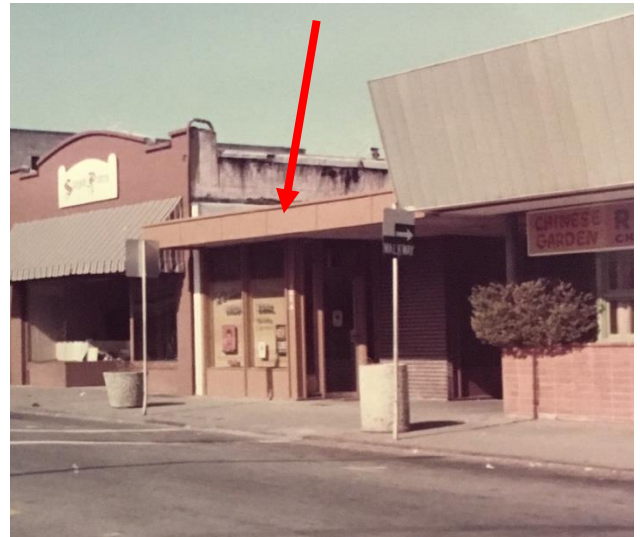
Above: Front façade before alterations.
