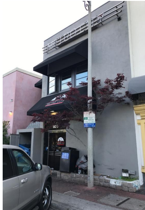
Above: Rear façade showing two stories.
