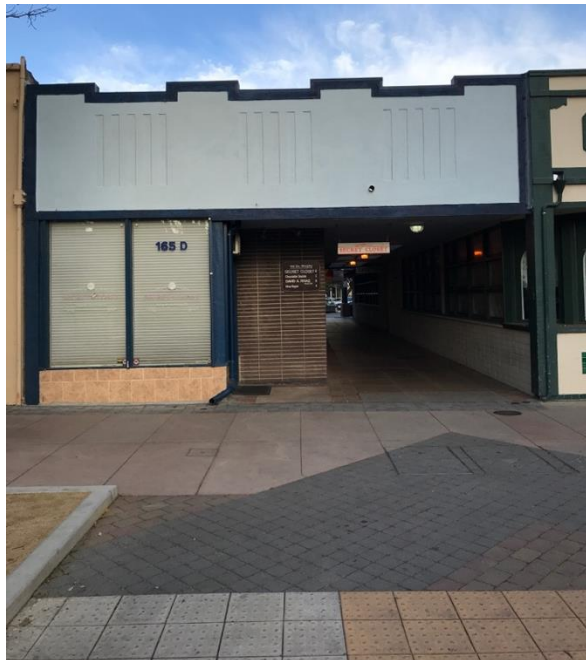
Above: Front façade showing relationship to walkway to parking lot.
