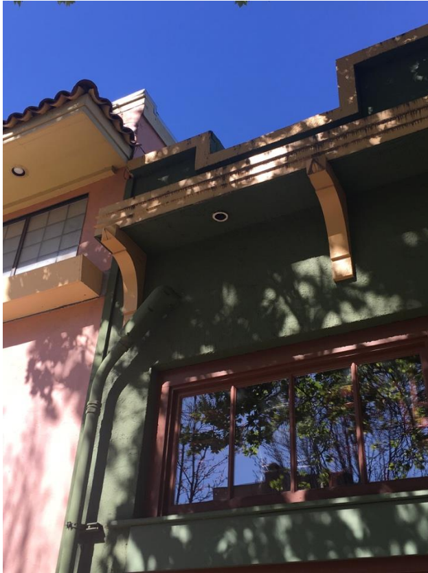
Above: Front transom detail and conduit on façade.
