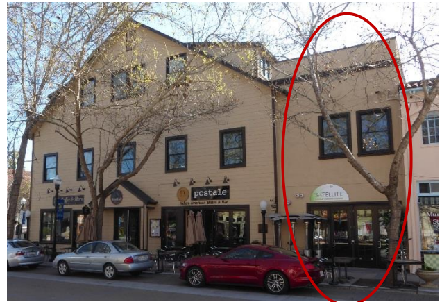
Overall building, Murphy Avenue elevation; circled area is later addition to the building.
