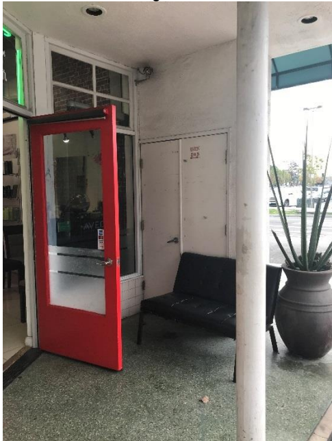
Below: Detail showing corner alteration
