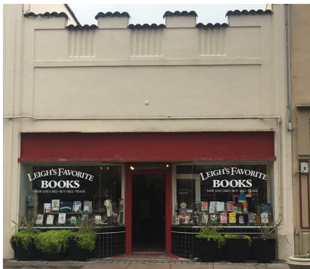
Above: The light color stucco makes the colored details like the black tile, awnings, and red tile capping stand out.
