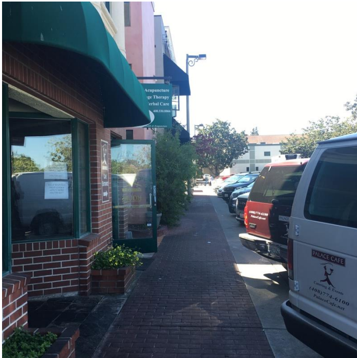
These rear facades of the west side Murphy Avenue buildings have a sidewalk, which helps with pedestrian safety. They also do not have any trash storage at the rear.
