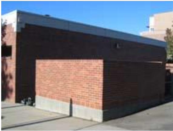
This trash enclosure in another commercial area was designed to blend with the existing architecture.
