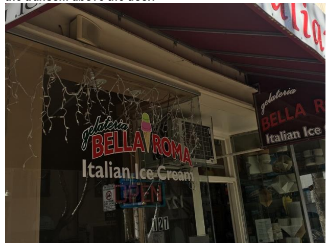
Below: This storefront has a window air conditioning unit in the transom above the door.
