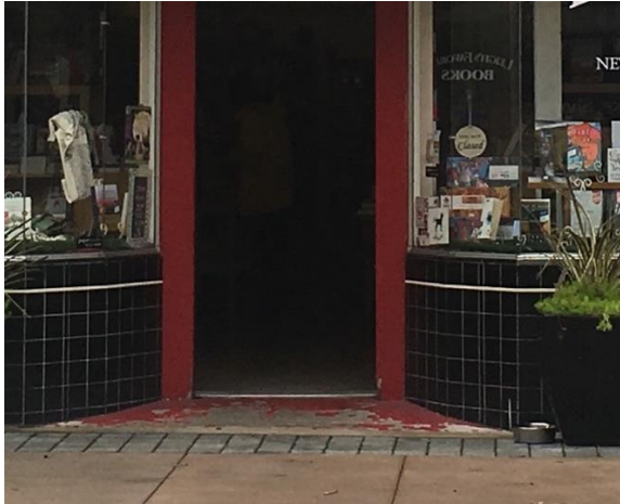
Above: Detail of recessed entry and tile work.
