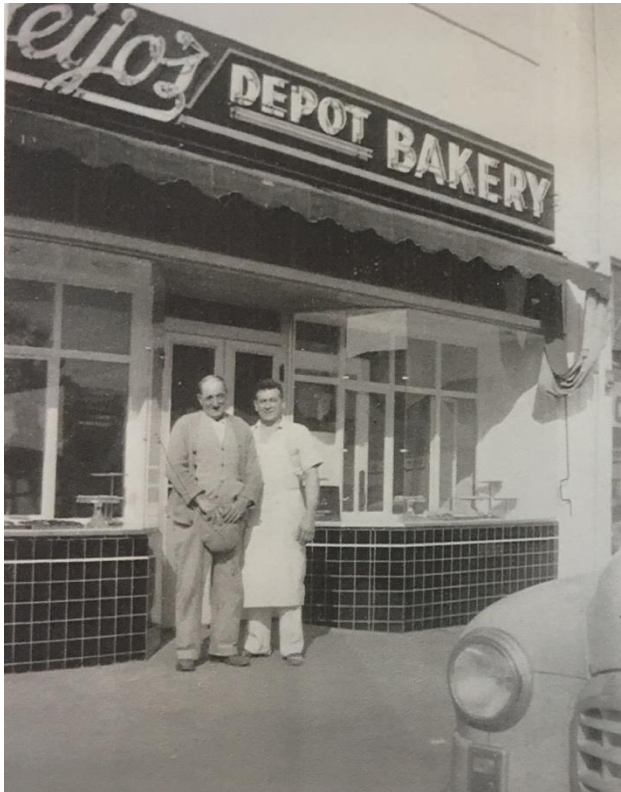
Above: An historic photograph showing the tile work below the window boxes.
