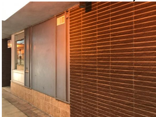
Below: Detail of Roman Brick in breezeway.
