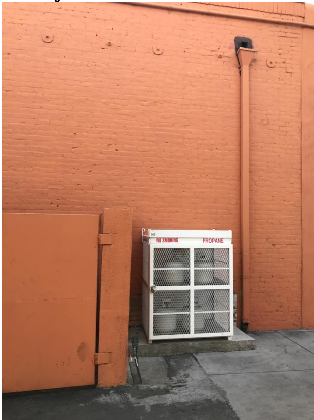
Below: The side elevation at the alley. Note the propane tank storage which is not recommended to continue.
