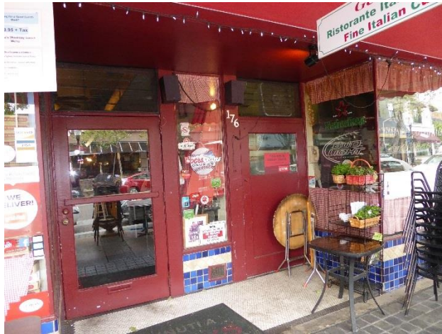
Above: Detail of entry doors.
