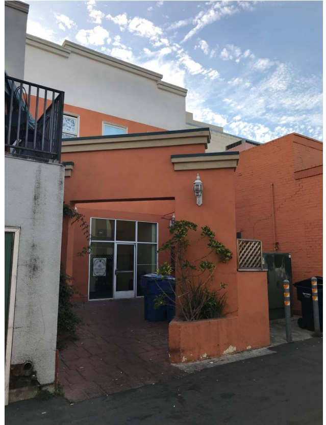
Above: Gateway to rear entrance.
