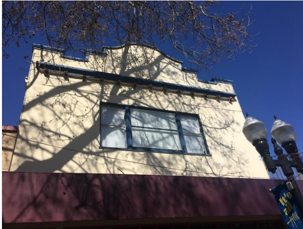
Above: Detail of the scalloped parapet at the Murphy Avenue elevation.
