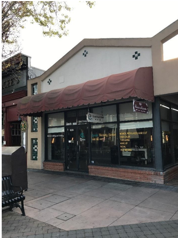
Above: One-story commercial building with storefront
