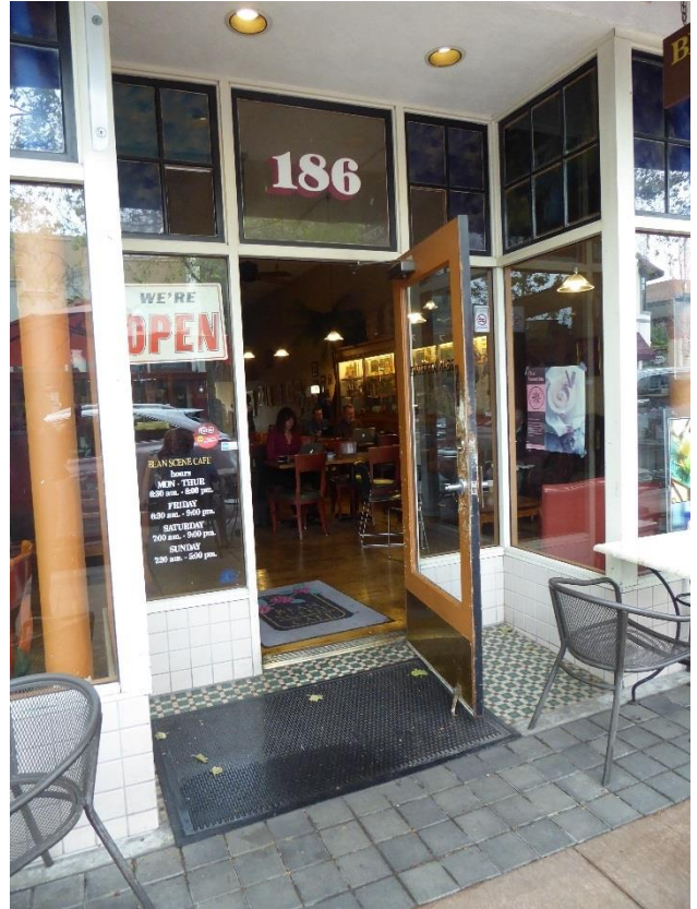
Above: Detail of typical restored storefront
