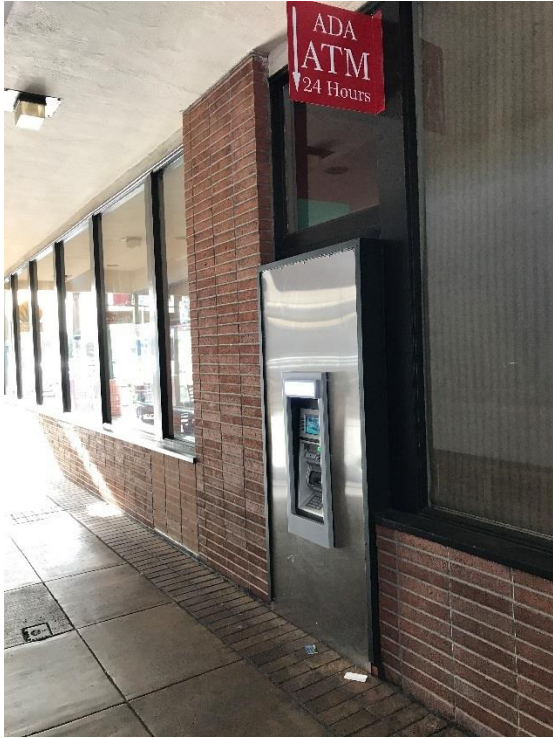
Above: Detail of the Roman brick that carries through the breezeway.
