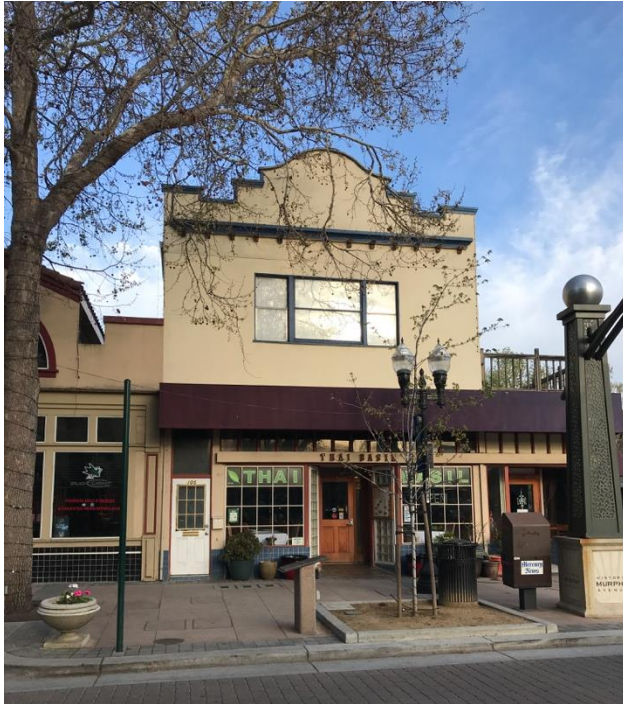
Above: View of this corner building looking west.
