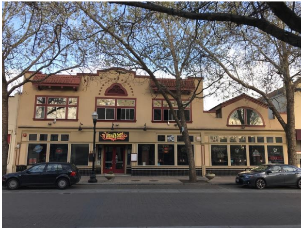
Above: View of the two-part façade, one and two story elements.
