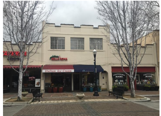
Above: Middle storefront with second story windows.
