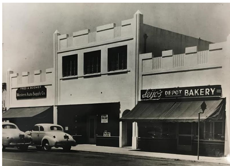
Above: Note the tile work at the storefront base, the stepped parapet, the signage area, and stucco finish at 121-133 S. Murphy Ave.
