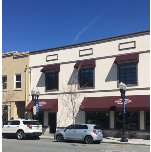
Above: The Washington Street elevation.
