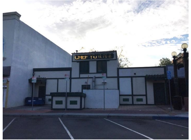
Above: Rear view showing trash area and adjacent parking.
