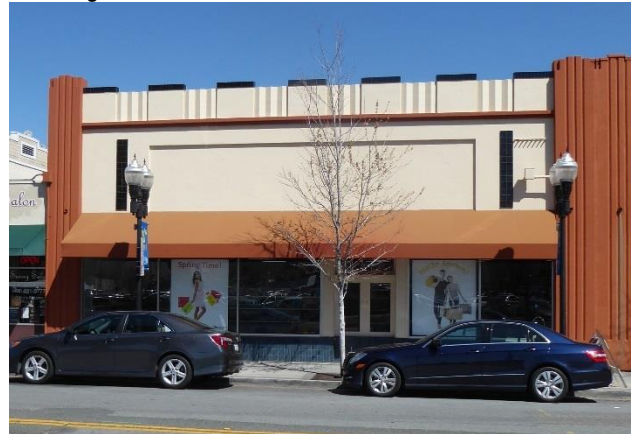
Below: 1940s portion of the building along East Washington.
