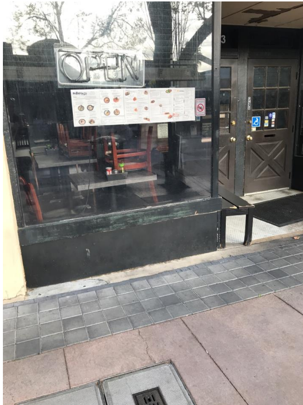
Above: Detail of the north side of the storefront.
