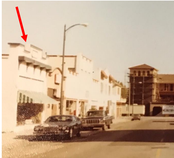
Above: 139 S Murphy c. early 1980s, building along Evelyn under construction.
