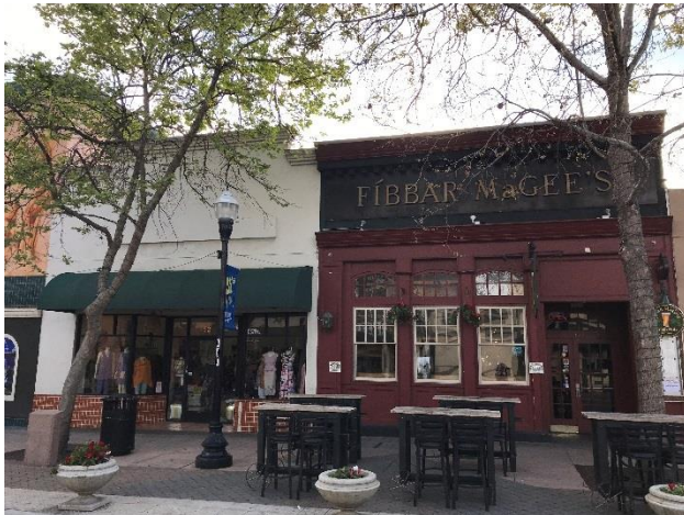
Above: Current configuration of this one-story commercial building with two storefronts.
