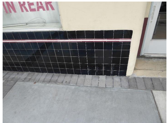
Above: Detail of tile base at storefront.
