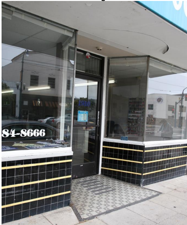
Above: An intact, recessed storefront from the late 1920s.
