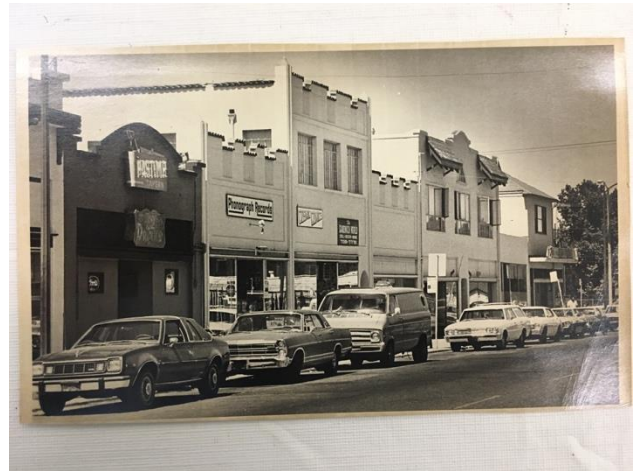
Above: A photograph of the building dating to about 1981, showing the addition of the red tile coping at parapet.
