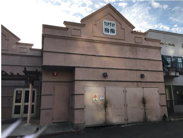
Above: Rear elevation with multiple doors.
