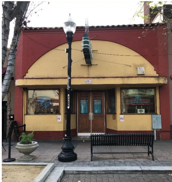
Above: One-story commercial building with Streamline Modern detailing at storefront
