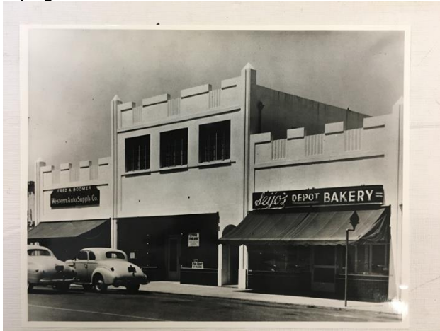
Below: The building just after construction, note no red tile coping at roof line.
