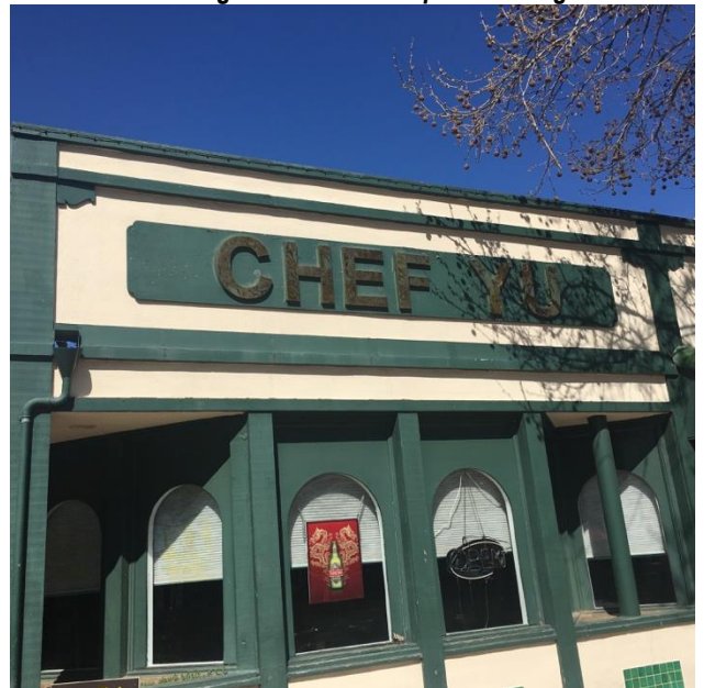
Below: Detail of sign band across top of building.
