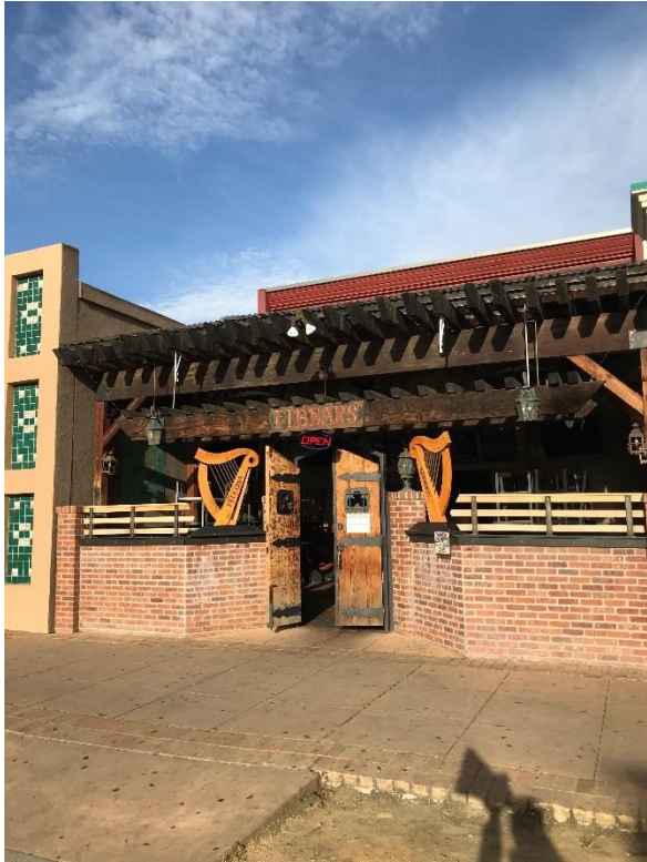
Above: Rear elevation of the north storefront.
