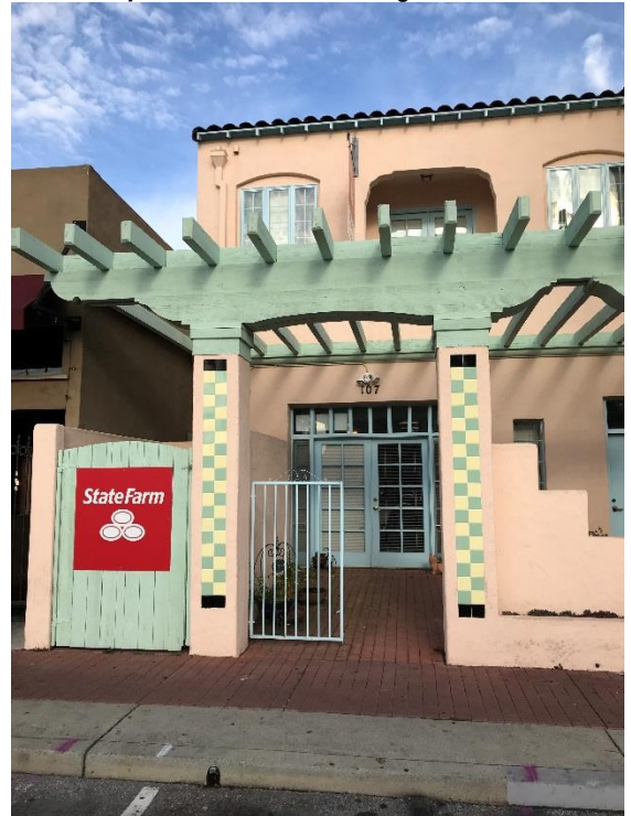
Below: Unpermitted State Farm sign on rear elevation
