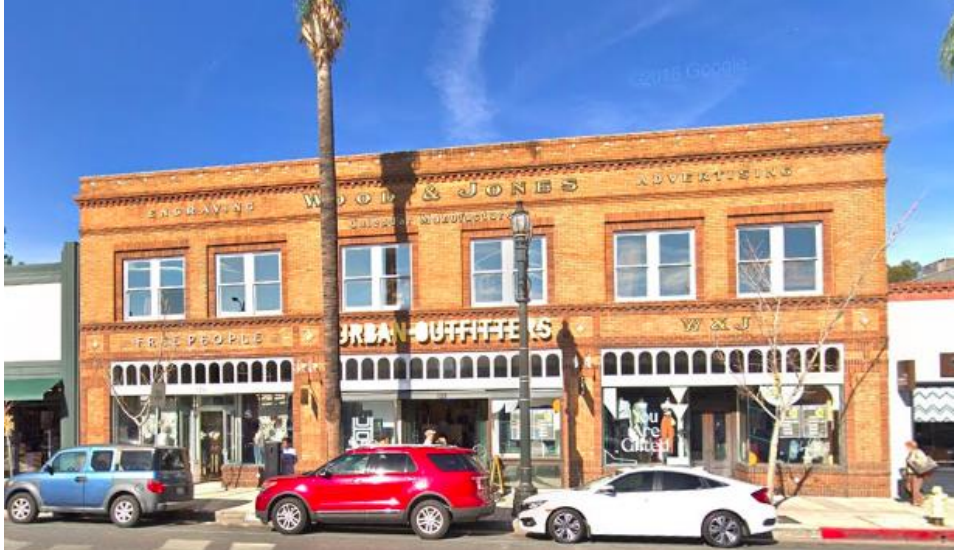
This chain store used simple applied letters as signage, respecting the established sign band and clerestory windows.
