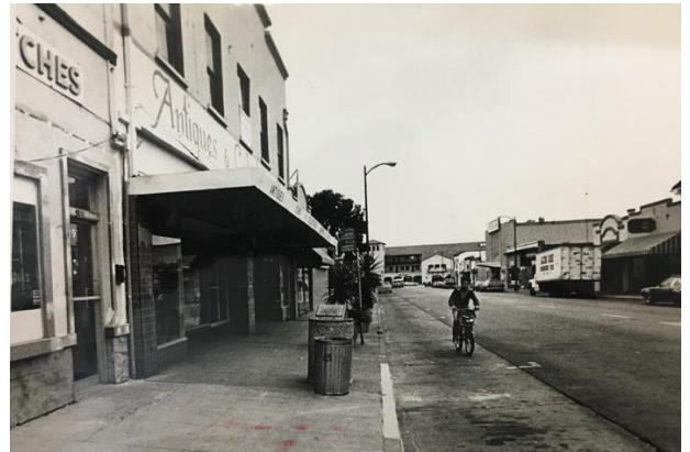
Above: View from the 1980s of the projecting canopy at Murphy Avenue.
