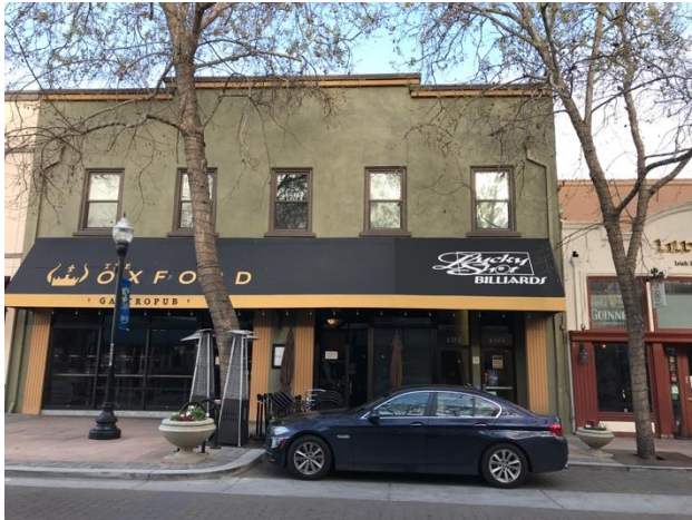
Above: Current view of the building.
