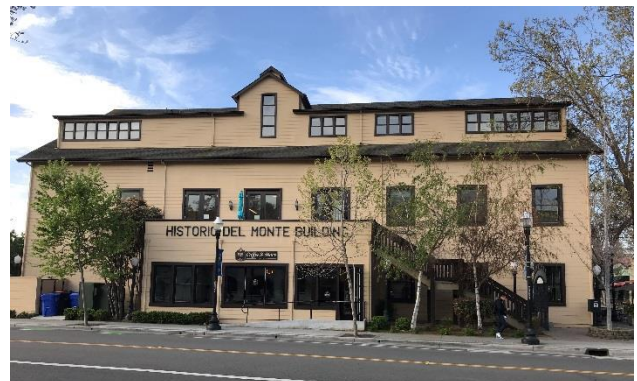
Overall building, Evelyn Avenue elevation.
