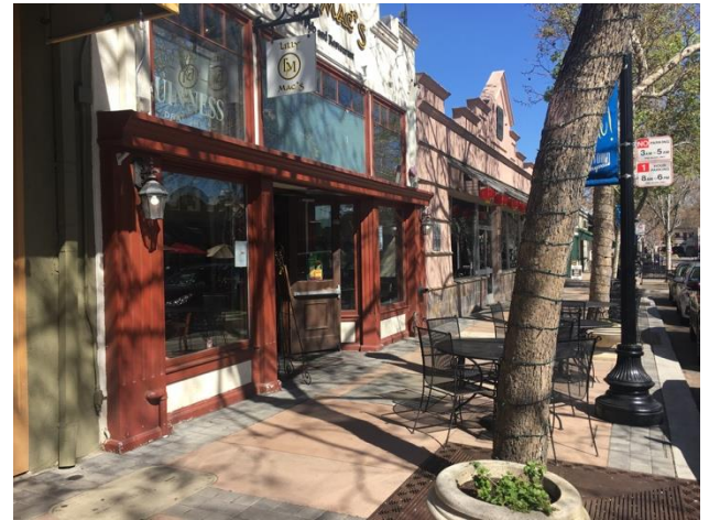
Above: The front storefront.
