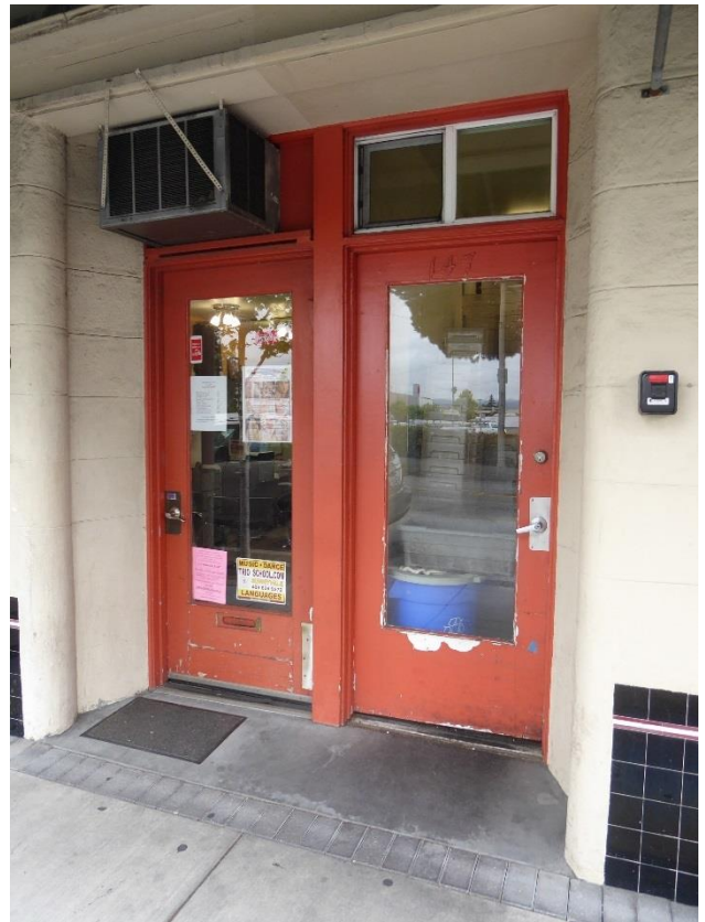
Above: Recessed entry with single panel glazed wood doors into the storefronts.
