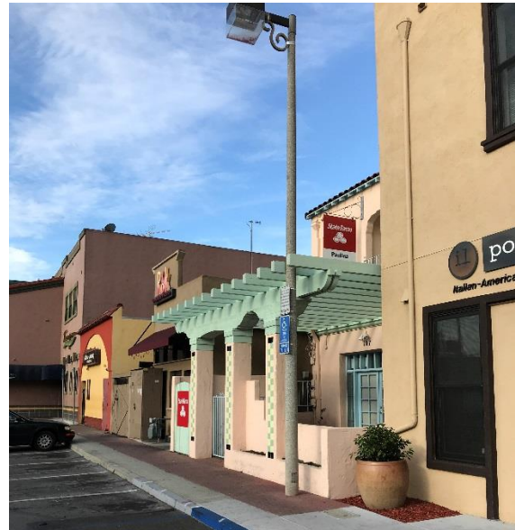
Above: Rear elevation from parking lot
