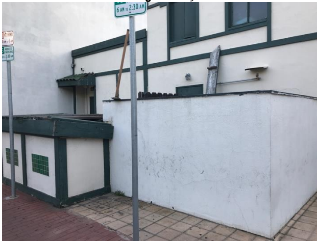
Below: Detail of the building rear façade.
