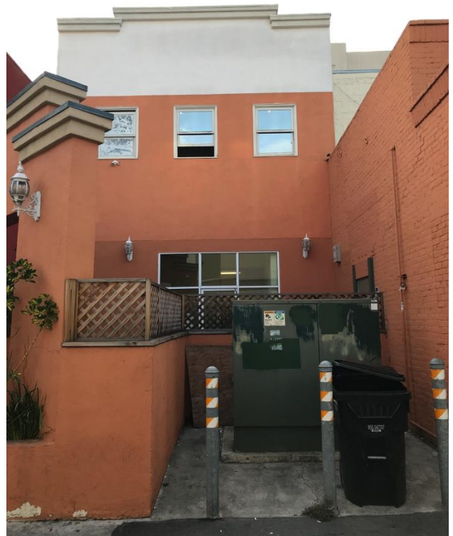
Above: Rear façade of building from alley
