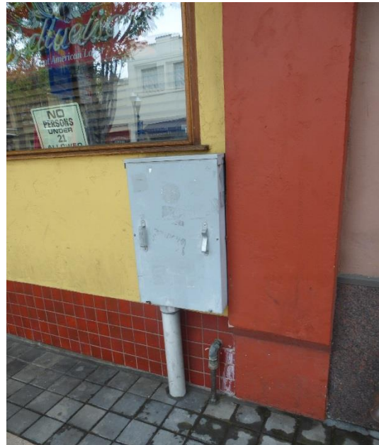
Above: Electrical box and conduit that distract from the buildings architectural features.
