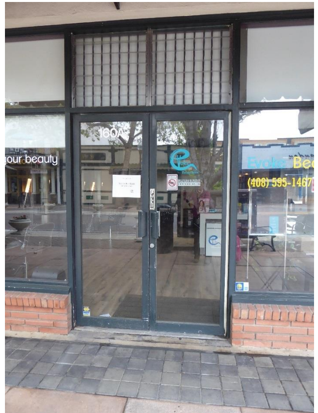
Above: Brick base, wood storefront windows and location of entry doors.
