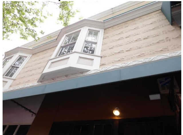
Below: Detail of bay windows and exterior finish
