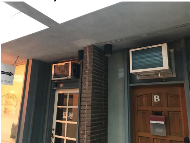
Below: Rear entry doors with air units above.
