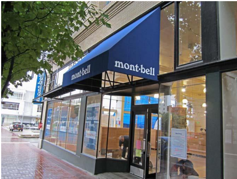
Above: This storefront is clearly modern but by employing a solid base, clear glass, well-placed and designed awnings and a blade sign at the corner, it will blend well with its historic neighbors.
