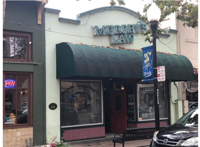
Below: Detail of the signage at the arched parapet.
