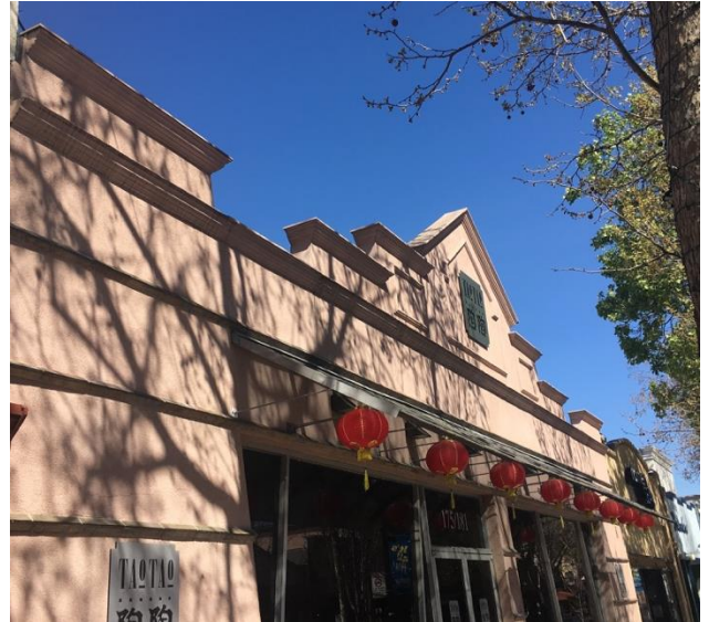
Above: Detail of overhang and roofline
