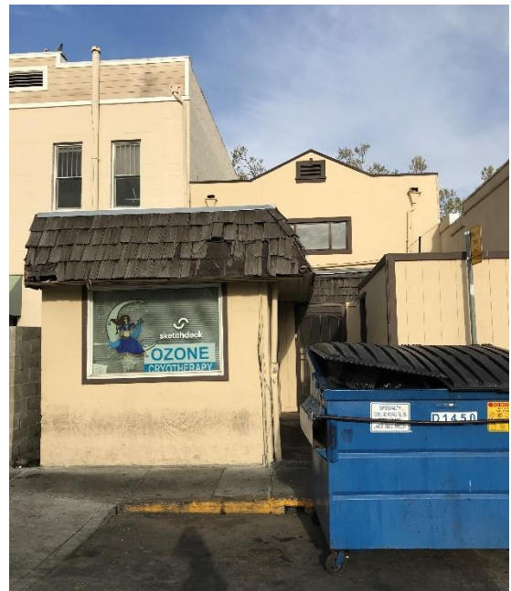
Above: Rear of storefront showing outbuildings and garbage dumpster.
