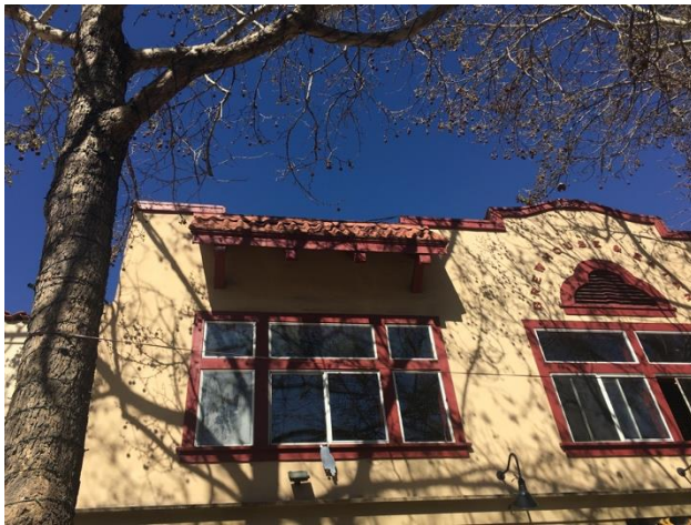
Above: Detail of windows, awning and decorative vent.
