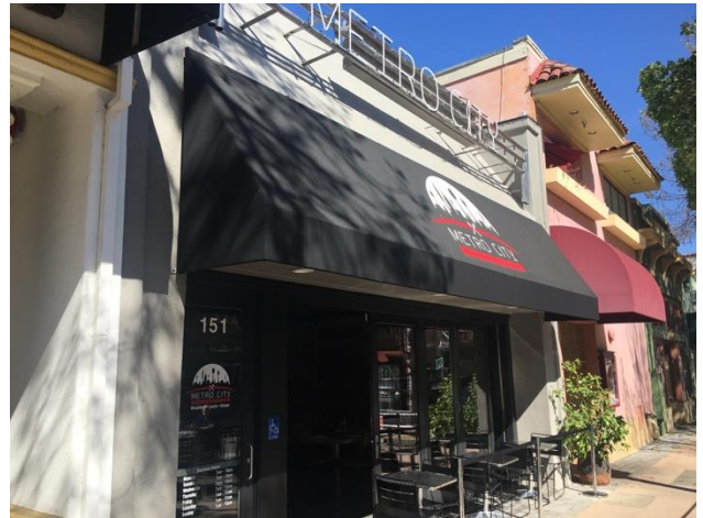
Above: Detail of the Murphy Avenue façade.
