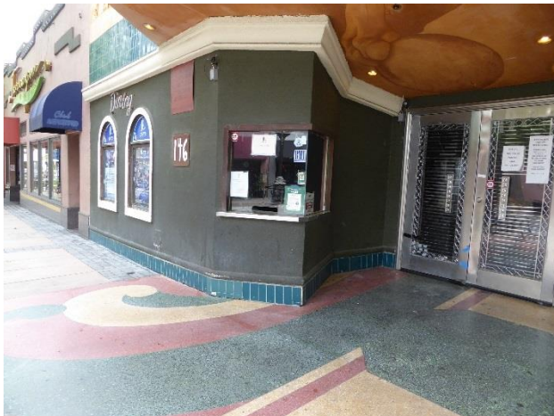
Below: Ticket window and terrazzo sidewalk.
