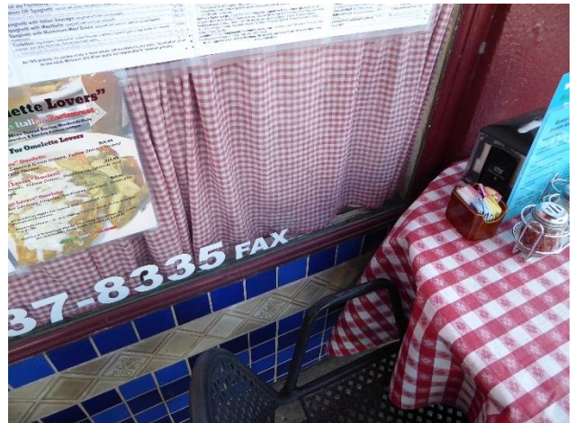
Below: Detail of ceramic tile base and metal-frame storefront window.
