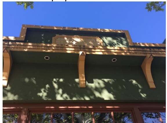
Below: Detail of parapet.
