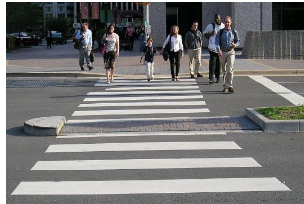
Example: High-visibility crosswalk and directional curb ramps
