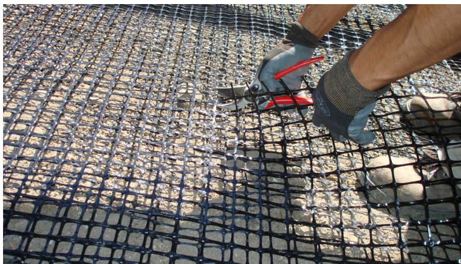
Biaxial Geogrid laid beneath patio, overlaid with drain rock
