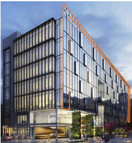
Figure 5. A free-standing glass "fin" extends along the margins of the building's north façade (shown in orange), posing a collision hazard to birds navigating around the building.
