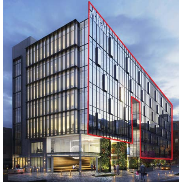
Figure 7. The proposed large expanse of glass on the building's north façade, while visually disrupted by narrow mullions and shadow boxes, will reflect the sky and nearby landscape vegetation, posing a potential collision hazard to birds.
