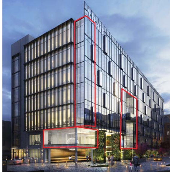
Figure 4. Examples of transparent glass corners (shown in red) at the building's northeast corner and at a recessed portion of the north façade. Additional transparent glass corners were identified at the building's northwest corner.
