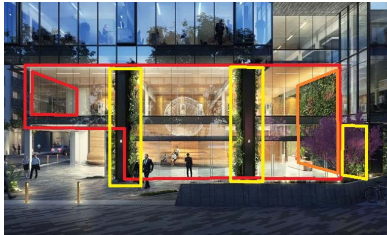
Figure 6. Birds may collide with glass surrounding the lobby at the transparent glass corner (red) or when attempting to fly in between exterior vegetation (yellow) and interior vegetation (orange).
