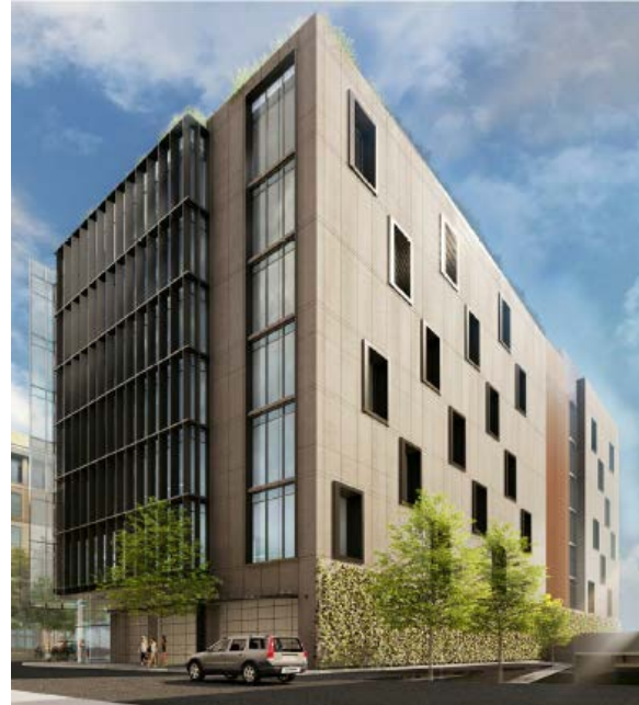
Figure 1. The building's west and east facades (the west façade is shown on the left) incorporate non-reflective fins that increase the visibility of glazed areas to birds, and the building's south façade (shown on the right) has limited glazing.
